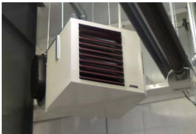
3: Gas fired Reznor unit heater adjacent to gas infra-red heater
