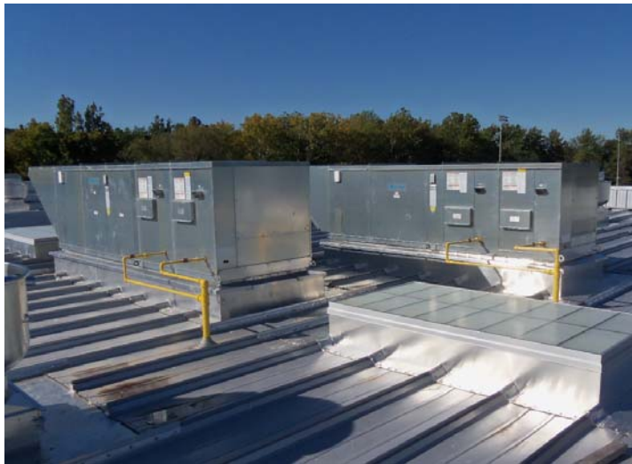
5: Two rooftop units (typical)
