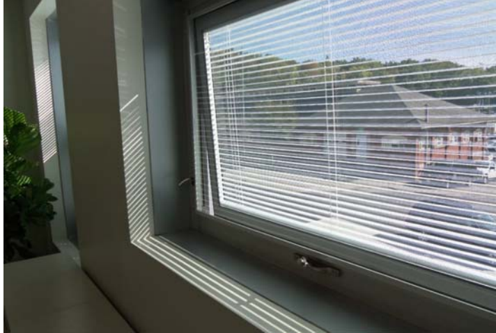
4: Window open while RTU providing conditioned air to space
